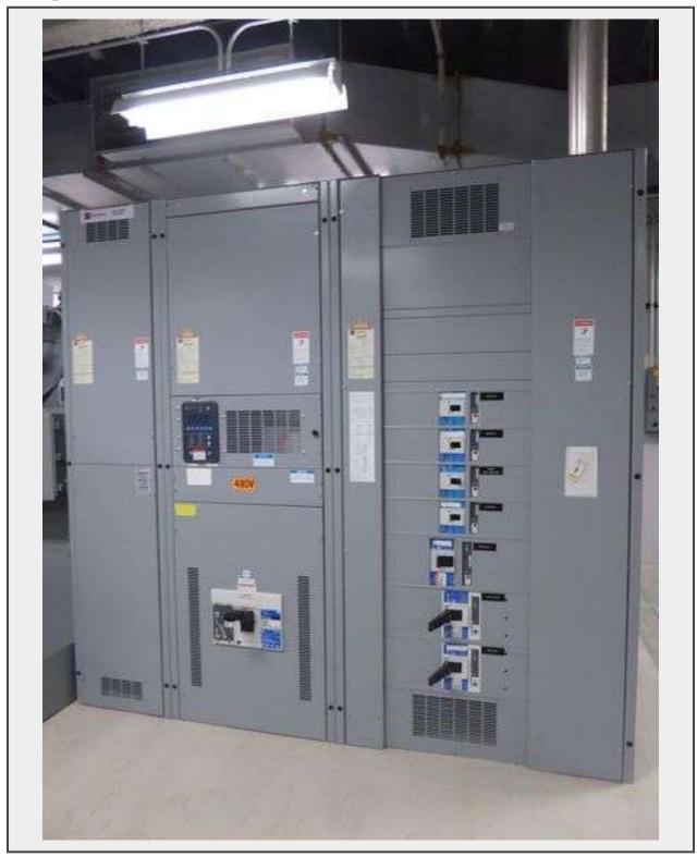
408Y/277V; (3) Vertical Sections Include: (1) 1600A Circuit Breaker; (4) 400A Circuit Breaker; (1) 600A Circuit Breaker; (2) 1200A Circuit Breaker; Tag: 275760 | Location: Chicago
